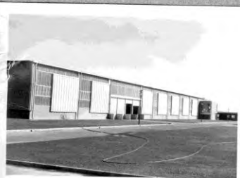
SOUTH SIDE OF MAIN STORES SHOWING LOADING AND UNLOADING BAYS.
